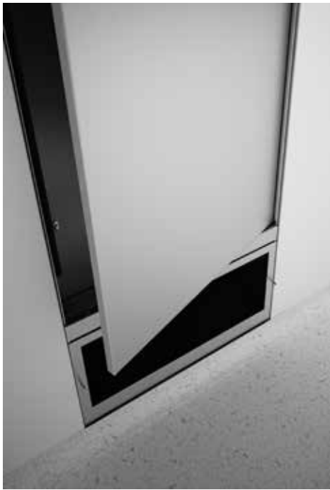
Exhaust air chute with inspection opening in combination with fibresept ventilation grille
