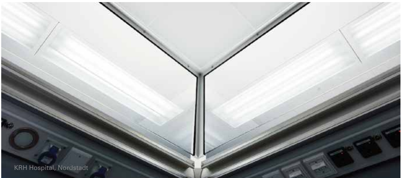
Clip ceiling system with circumferential strip lights and connection to low-turbulence displacement flow panel.
