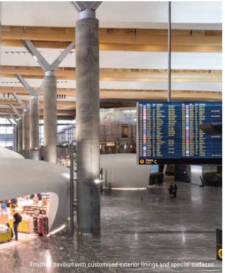
Finished pavilion showing customised interior metal cladding following the individual organic shape of the pavilion
