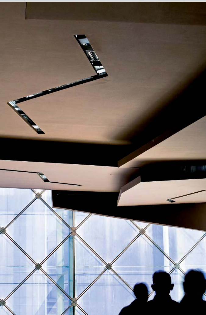
Metal ceiling panels in the foyer
