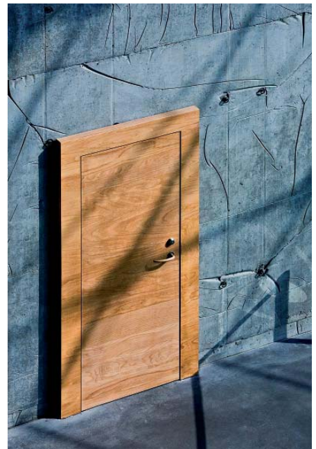
Exposed concrete wall with fire resistant wood door
