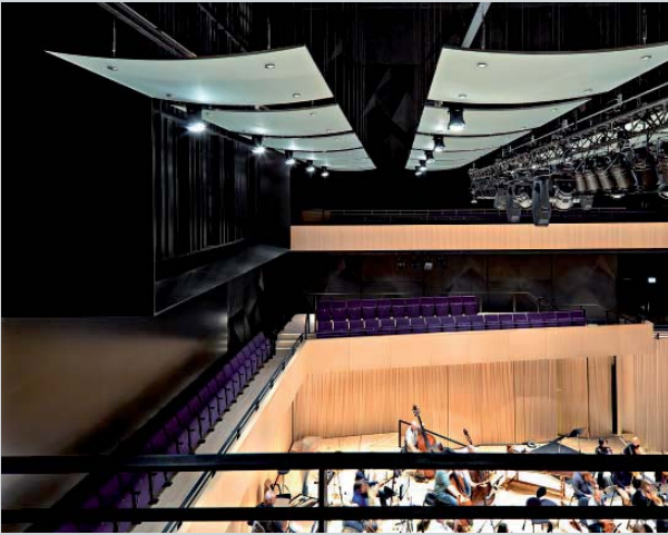
Bended ceiling reflector with heat strengthened frosted glass
