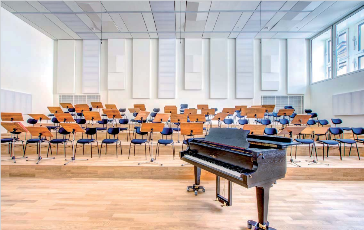
Rehearsal room with acoustically effective wall and ceiling panels
