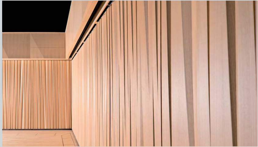
Vertically milled wall cladding with ash surface in concert hall
