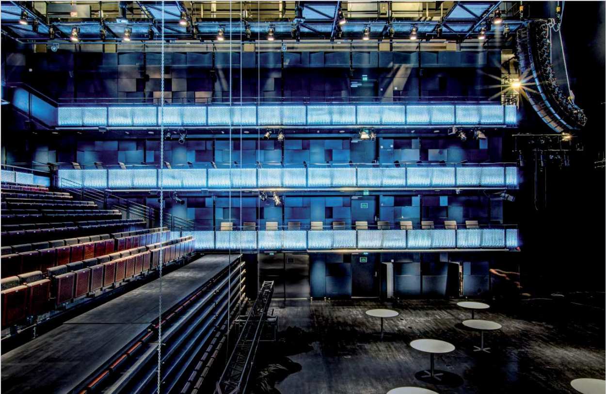
Multi-purpose hall with expanded metal balcony fronts
