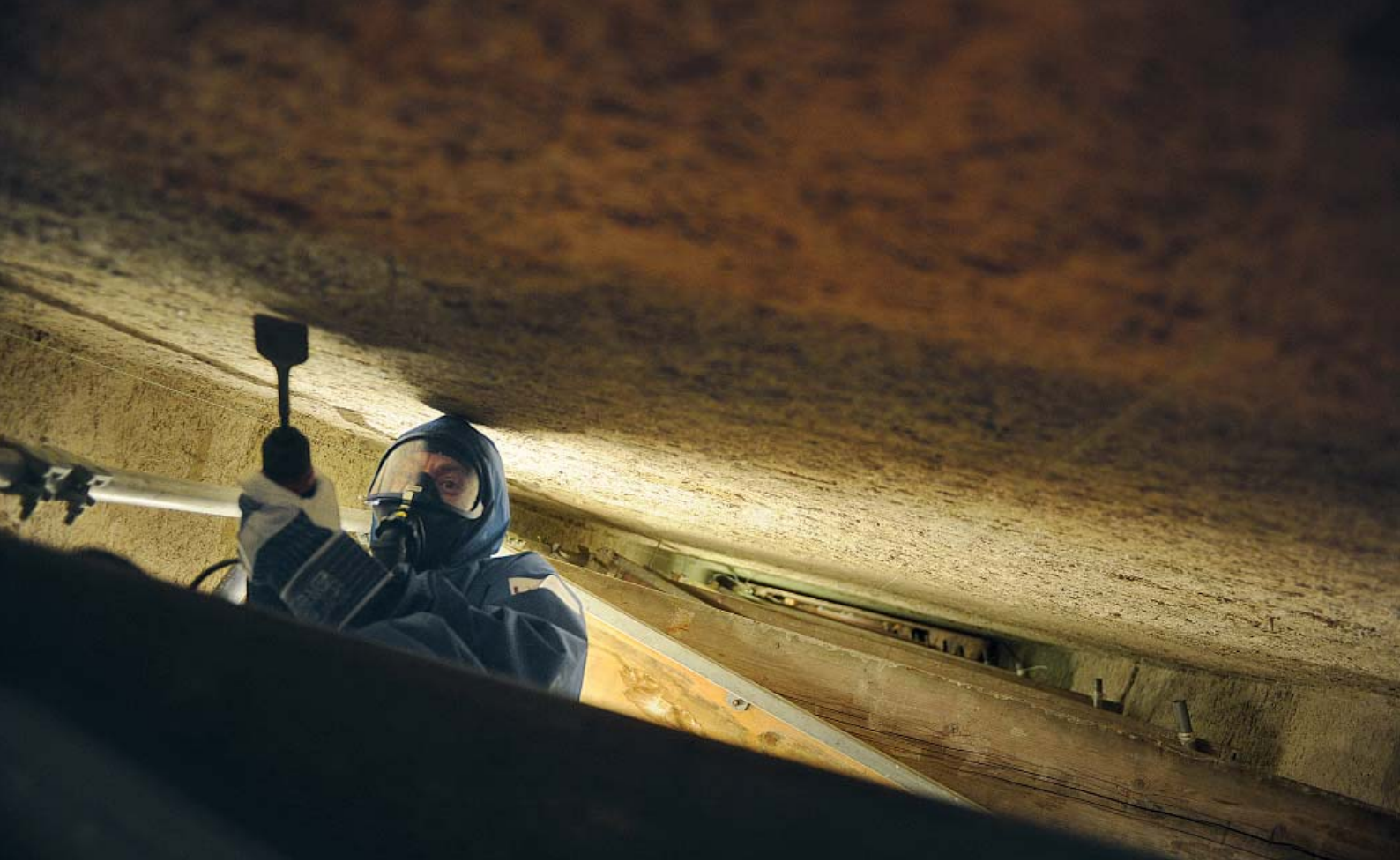
Renovation of contaminated plastering in maintenance shafts
