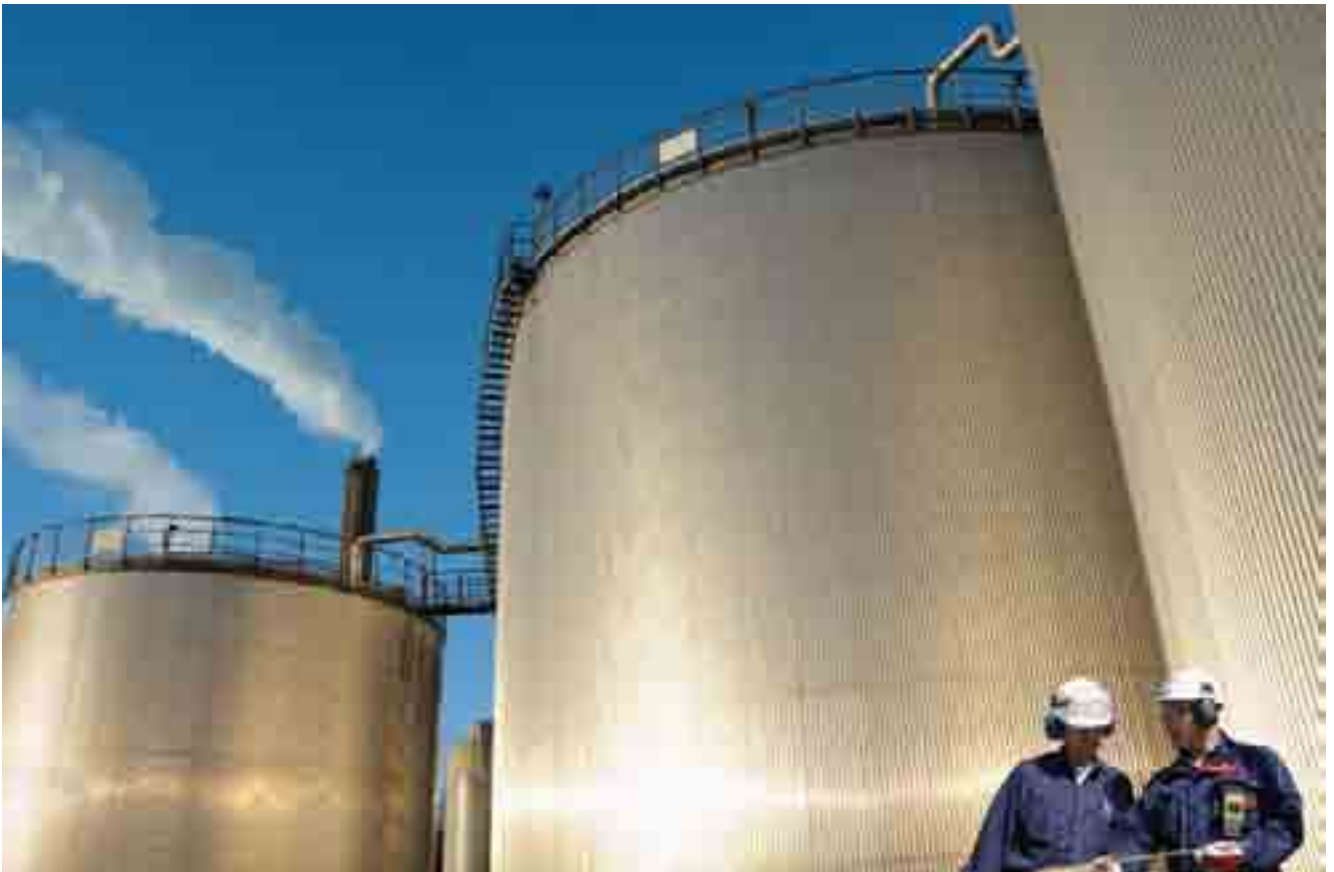
Oil tank insulation with profiled sheeting in Great Britain
