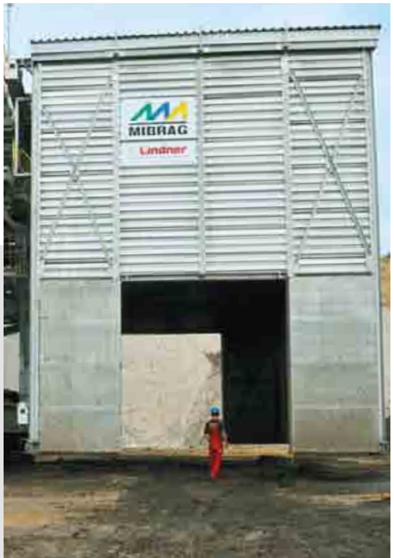
Sound insulation cover, lignite opencast pit in Schleenhain
