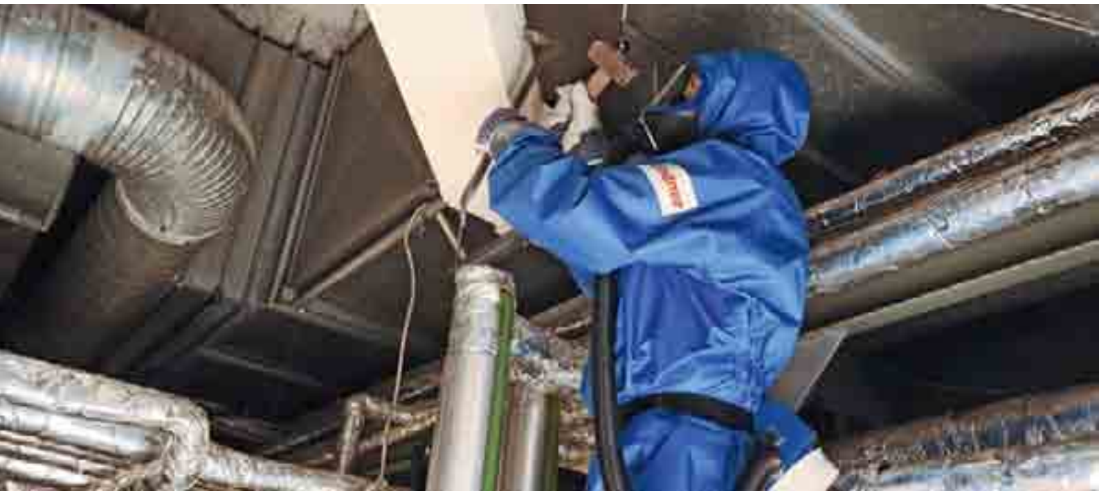
Removal of an air duct containing asbestos
